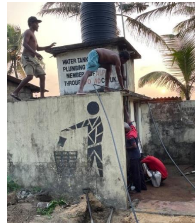
Fixing the water tank
